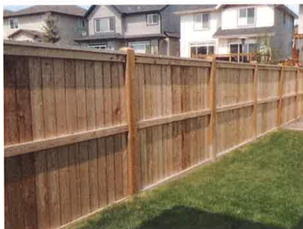
Figure 3-5 – Typical Neighborhood Fencing
