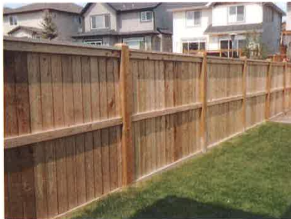
Figure 3-13 – Typical Neighborhood Fencing
